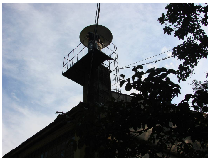
Figura 4.6 – Antena da Professional HRPT SMART Station Instalada no CEPSRM
